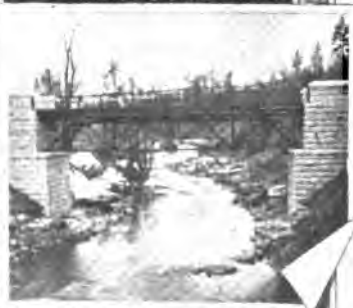
HIGHLAND CREEK BRIDGE
